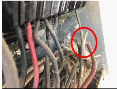
Disconnected wires in panel.
