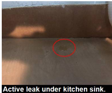
Active leak under kitchen sink.
