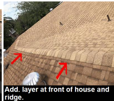
2 visible layers at front porch.
