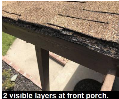
2 visible layers at front porch.
