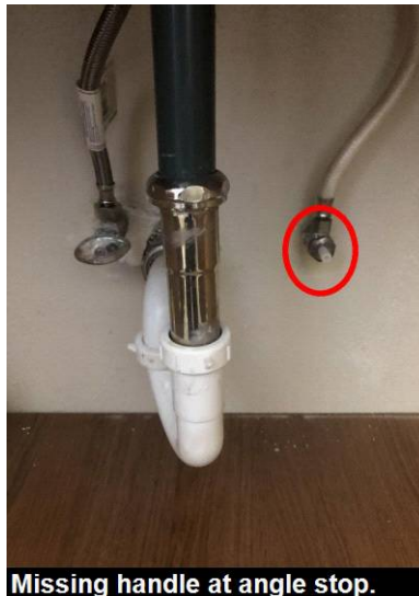
Missing handle at angle stop.
