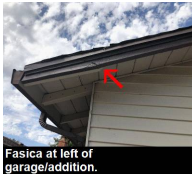
Damage at eave.
