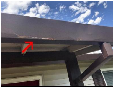
Rust at gutter over entry.
