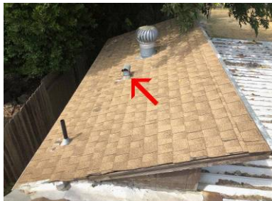
Rusted flue pipe.
