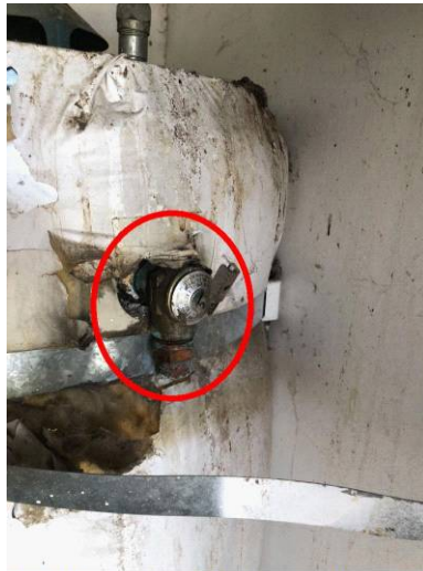
TPRV missing discharge line.
