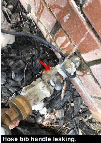
Hose bib handle leaking.
