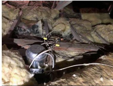
Inconsistent insulation levels.
