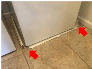
Damaged drain pan
