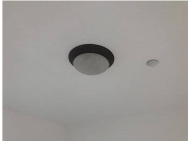
Fixture in bedroom #1
