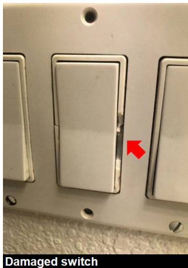
Damaged switch
